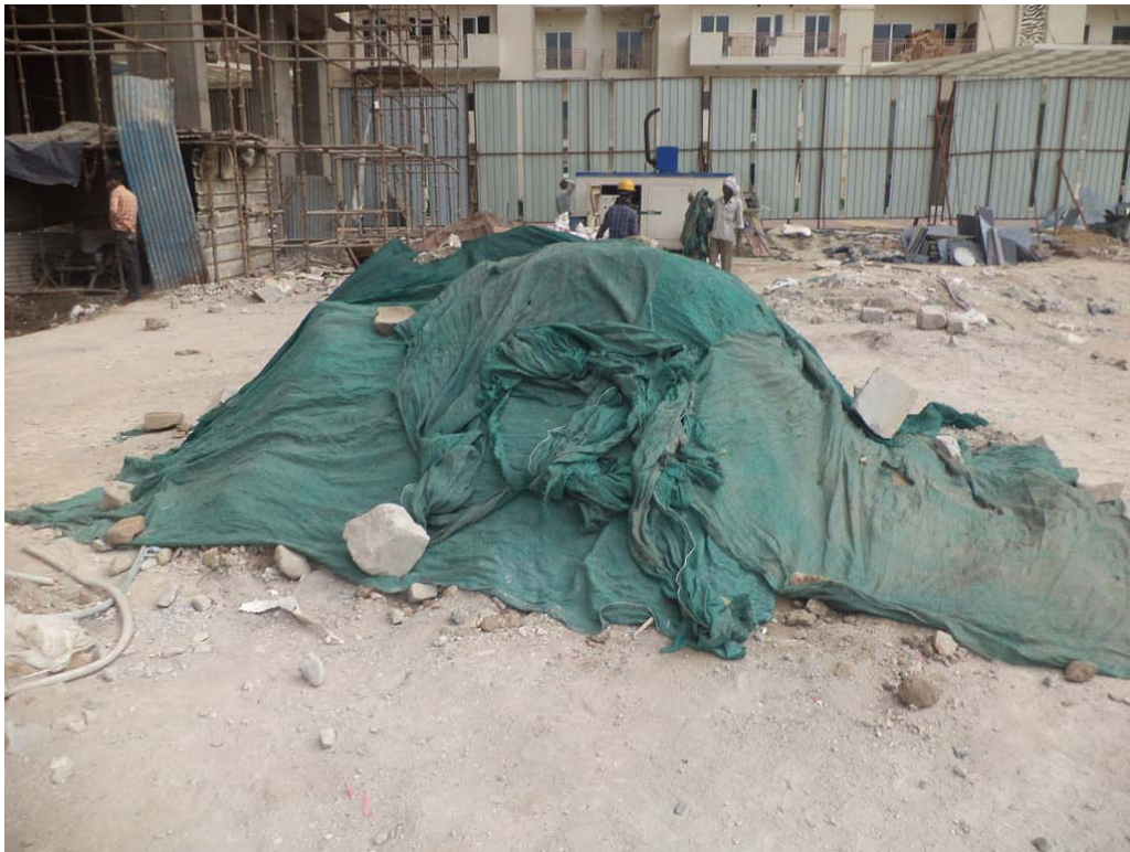
Covered Construction Material
